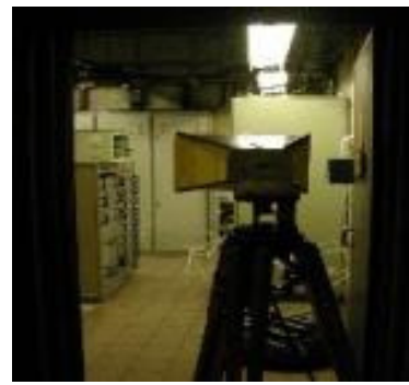
EMC Testing in Communication Room
